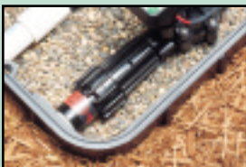
3/4" In-line 30 psi pressure regulator
