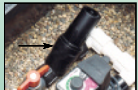
3/4" In-line "Y" filter with 200-mesh screen
