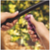
Insert emitter into 1/2" drip tubing
